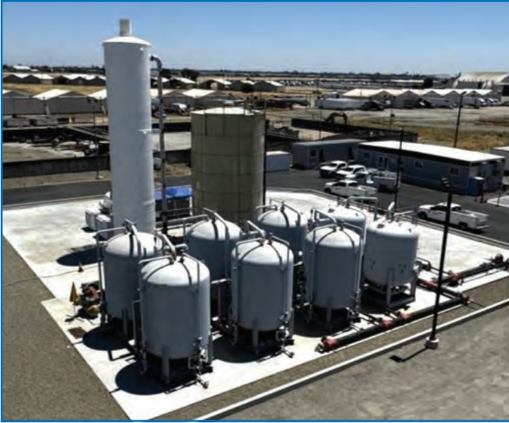
Above drone photo showing the new McClellan groundwater treatment plant constructed in 2024. Foreground shows 8 granular activated carbon vessels that can be utilized for additional groundwater treatment.
